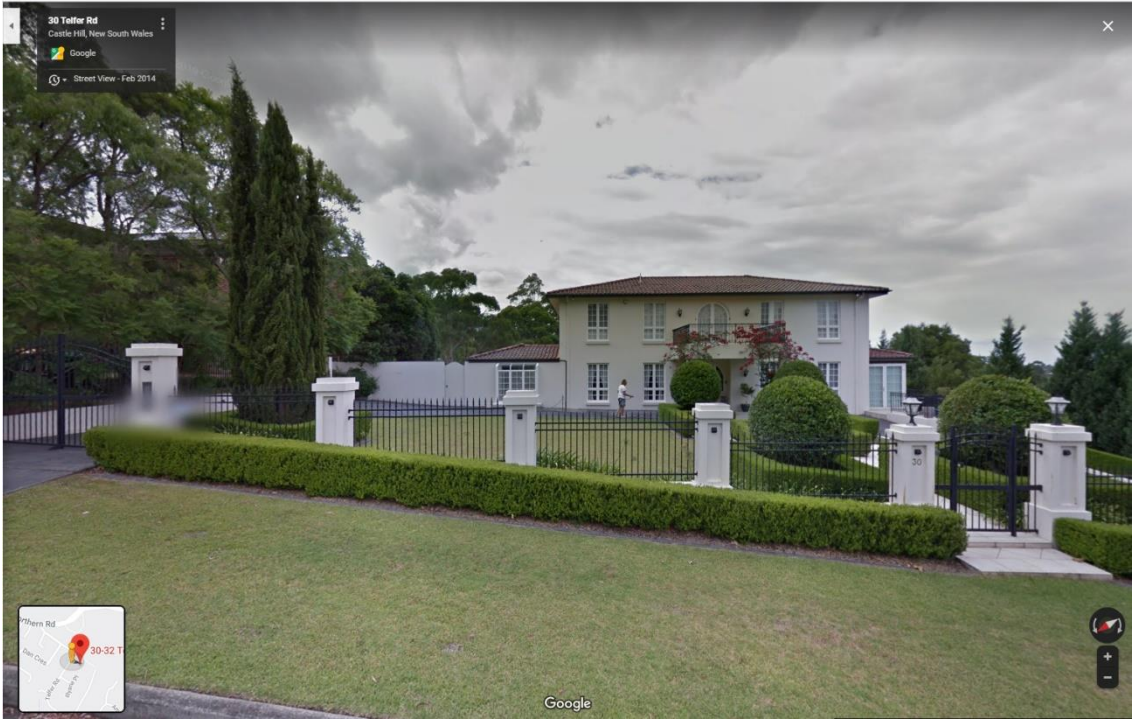
View of the dwelling, looking east
